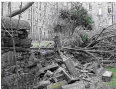
Collapsed freestanding wall from SCOTCROSS
