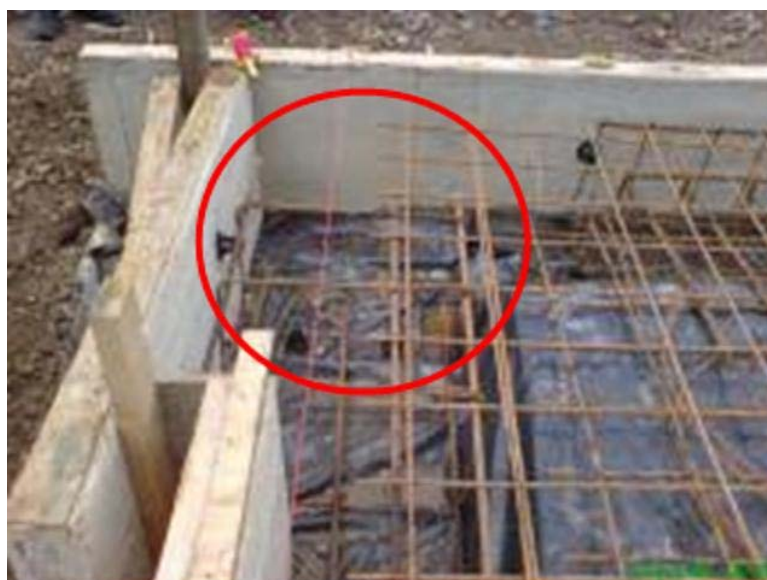
Missing reinforcement
