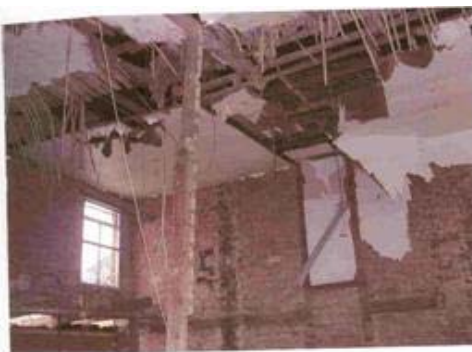
A 'prop' spliced together from old floor joists
